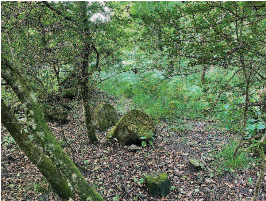
Photograph 2: Remains of Cannop Stone Works in the northern part of the site
