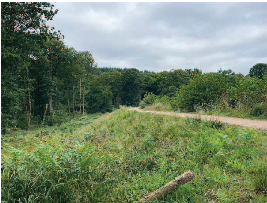
Photograph 11: Upper Cannop Pond embankment
