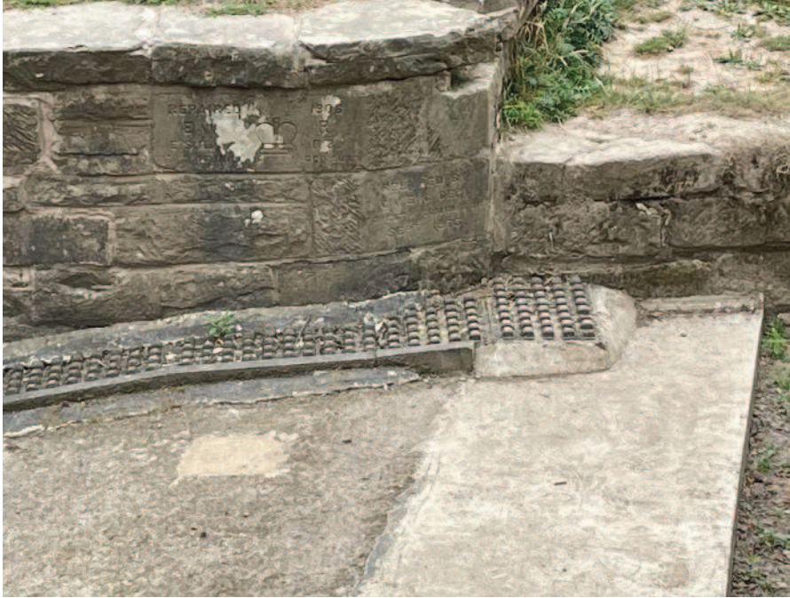
Photograph 9: Records of works carved into the stonework at Lower Cannop weir
