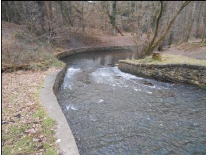
Spillway channel.
