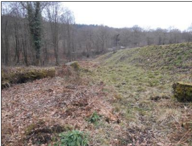
Downstream toe area.
